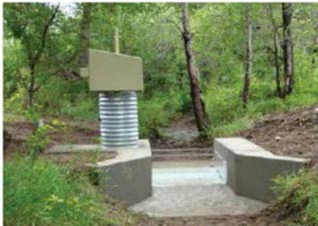
This Acequia Madre de Los Vigiles Flume at Rio Gallinas (left) and the lower staff gage (right) are two types of water flow measuring devices used to measure the flow of the water that goes through them or over them. The public, as well as OSE/ISC staff will soon be able to easily access a growing set of real-time water flow measurement data collected in various river basins.
