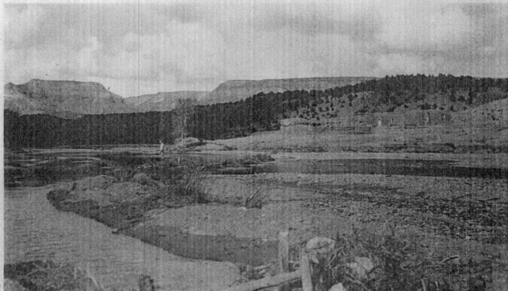
No. 10. Diversion Dam in Jemez River, and acequia Molino leading therefrom.
