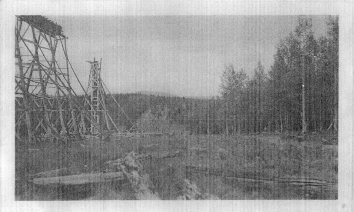
No. 13. The old flume and pressure pipe for the ditch taken out of Red River and used for placer mining near Elizabethtown in the Canadian River drainage.
