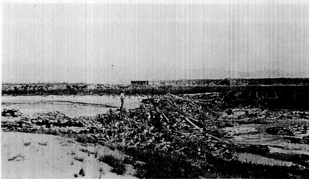
No. 48. Diversion Dam on the Rio Puerco near Cuba. Made of cedar trees typical of Rio Puerco.
