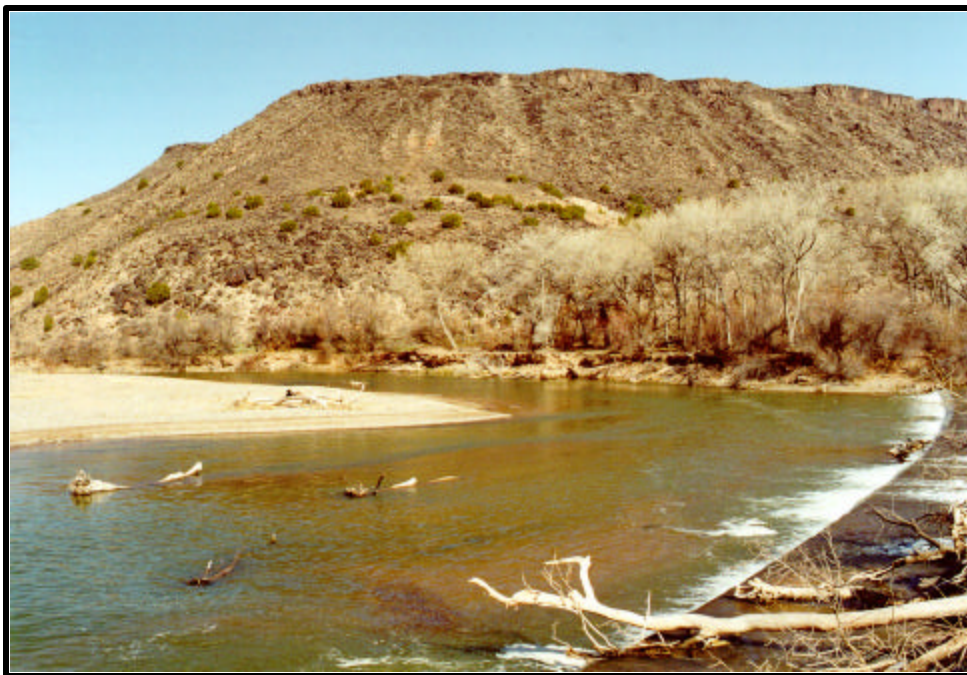
Plate A.8. View of Rio Grande at the Angostura Diversion Dam at RM 209.7. Note a bank height of about 6 to 8 feet, indicating some channel degradation below the diversion.
