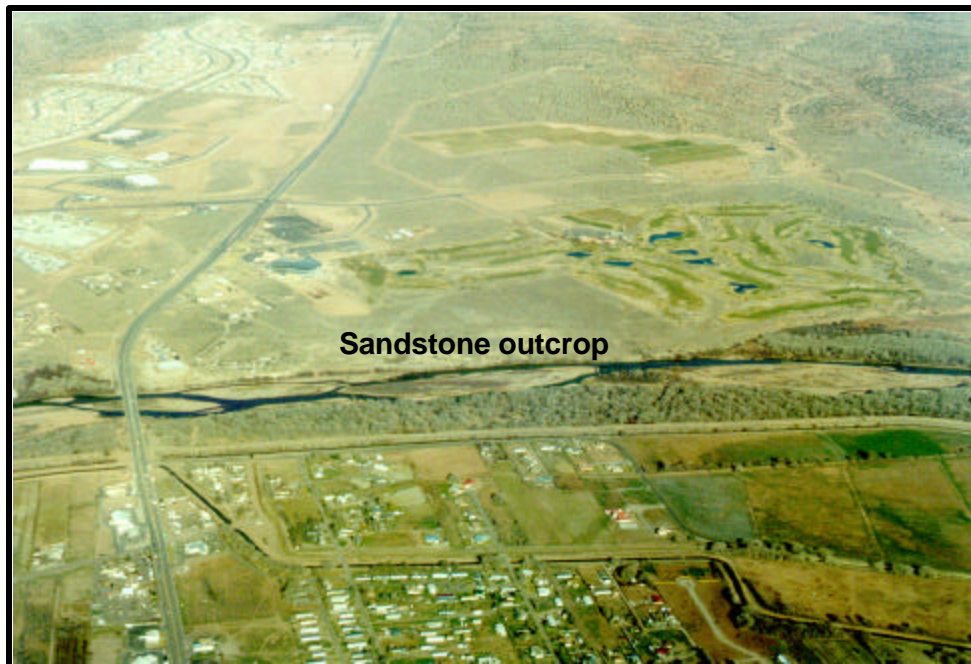
Plate A.10. View of Rio Grande at Highway 44 Bridge at Bernalillo (RM 204). The Coronado State Monument is located along the right bank, and it is at this location that sandstone outcrop in the Santa Fe Formation prevents westward migration of the river. Note the partially vegetated sand and gravel bars in the channel.
