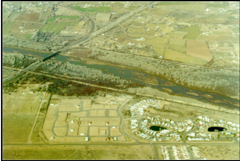
Plate A.17. View of Rio Grande in the vicinity of the BNSF Railroad bridge at Belen (RM 147.7). Note the numerous braid bars in the channel. This is the boundary between geomorphic Subreaches 4a and 4b.
