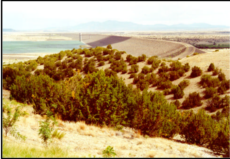
Plate A.1. Cochiti Dam at about RM 232.
