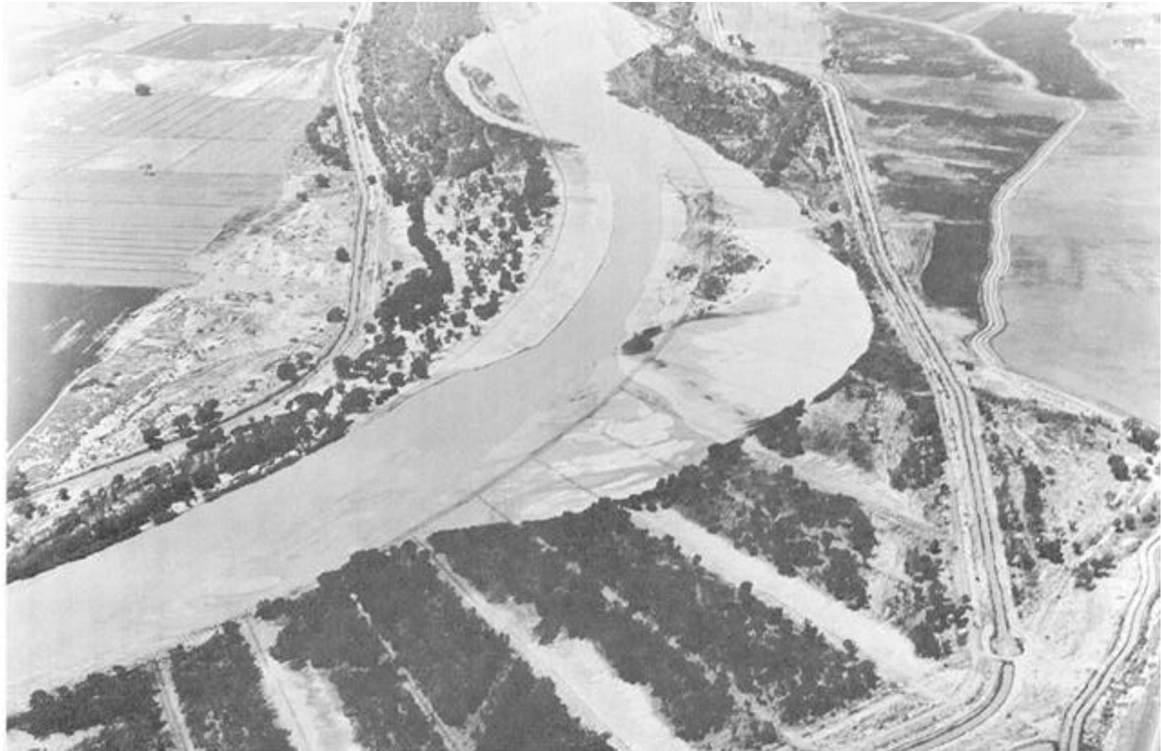
Figure 3.82. Aerial view of a completed jetty system, including a dredged pilot channel on the Middle Rio Grande (COE, 1963).
