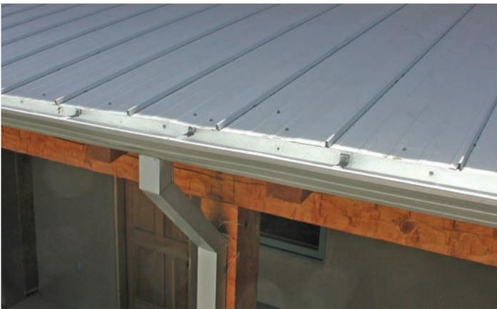
Figure 8-1: Gutters collect water from a pitched metal roof.
