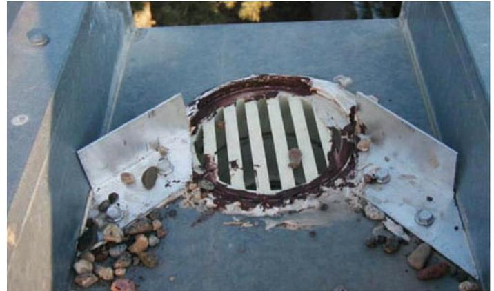
Figure 8-6: Partial dams installed on both sides of a drain directs the flow of rainwater.
