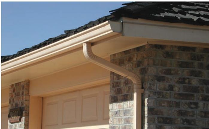
Figure 8-3: Photo of a downspout. Downspouts funnel water from gutters along a vertical drop.
