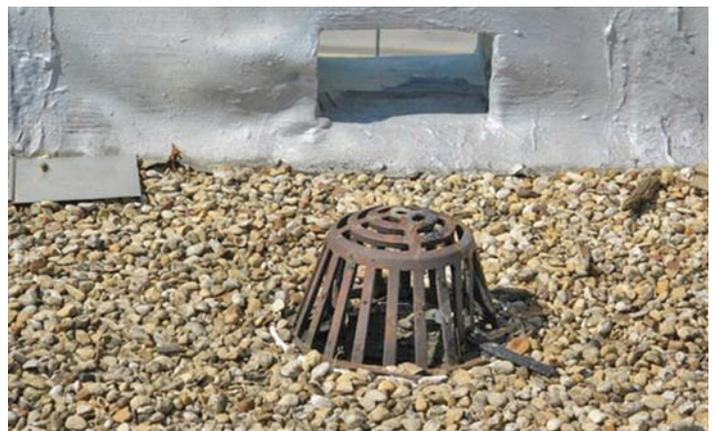
Figure 8-2: Photo of a roof drain. Note the canale opening, which is required for secondary drainage.
