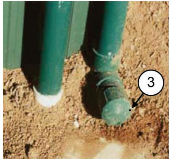
Figure 8-12. The cap on the first-flush pipe has a small hole drilled in the cap. Positioning the hole at the “3 o’clock” position enables water to slowly drain from the pipe while leaving sediment behind. The cap can be unscrewed for cleaning out the sediment.
