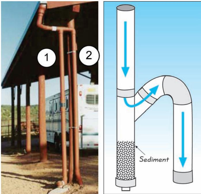
Figure 8-11. Roof water is initially conveyed from the downspout into a pipe (#1) that dead-ends (preferably near a planting bed). After that pipe fills, the cleaner water flows through pipe #2 to a cistern. The cutaway illustration shows how sediment settles in the first pipe.
