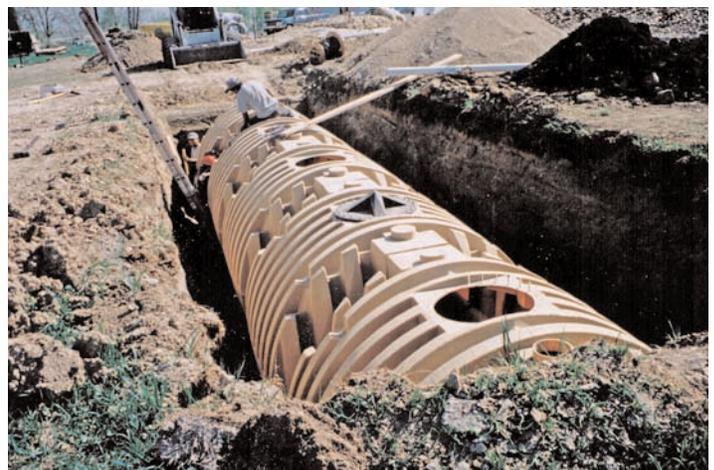
Figur 9-2: An underground cistern being installed.
