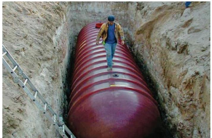
Figure 9-9: A fiberglass tank being installed.
