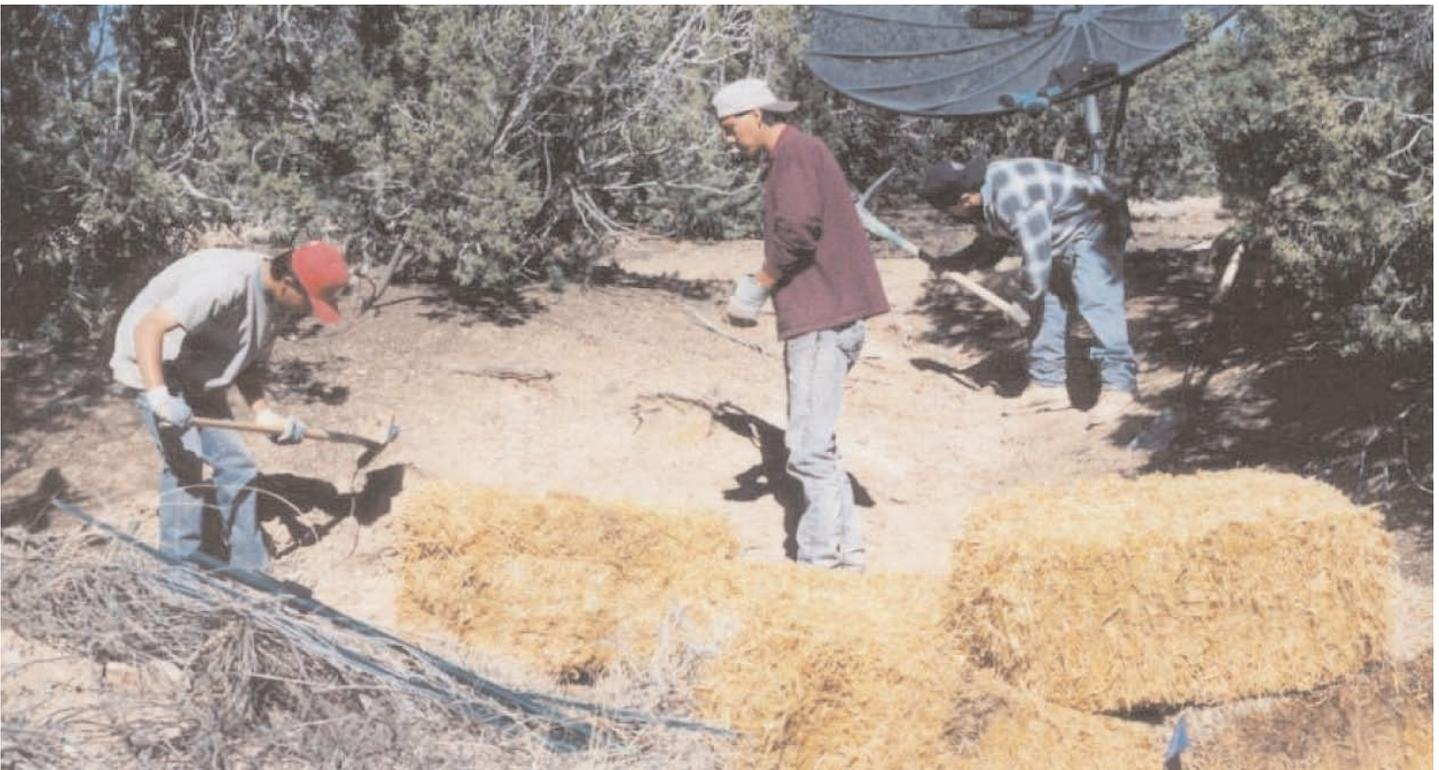
Figure 1-4: Workers install a straw bale swale.
