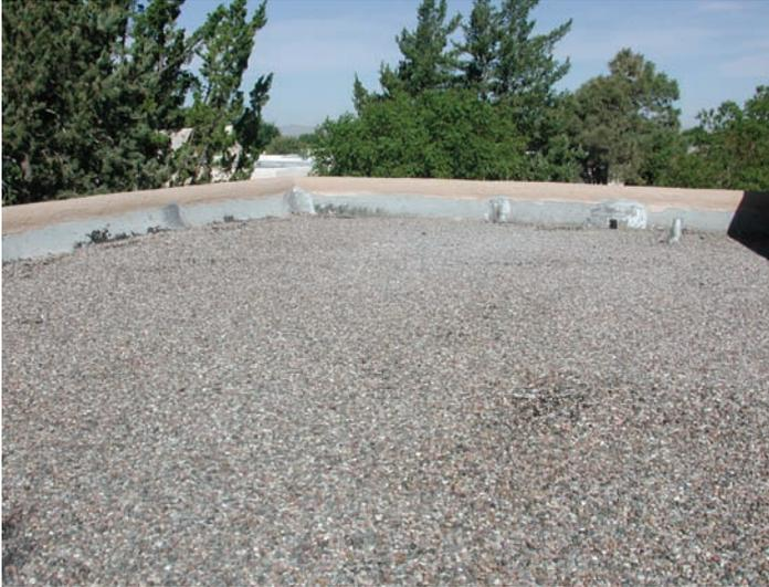
Figure 7-2: Although not the most efficient surfaces for harvesting rainwater, flat roofs can serve well as catchment areas for roof-reliant landscaping systems.
